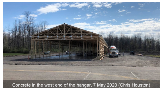
Concrete in the west end of the hangar, 7 May 2020 (Chris Houston)
