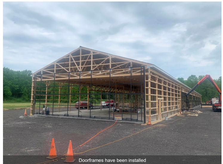
Doorframes have been installed
