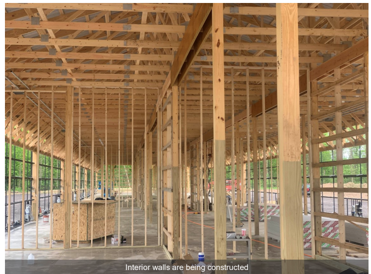
Interior walls are being constructed
