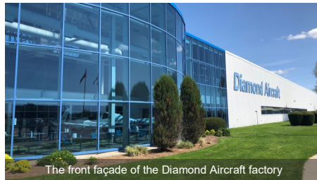
The front façade of the Diamond Aircraft factory
