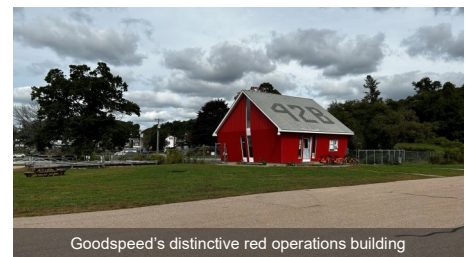
Goodspeed's distinctive red operations building
