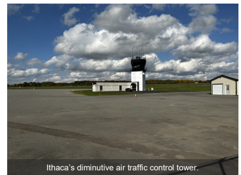
Ithaca's diminutive air traffic control tower.
