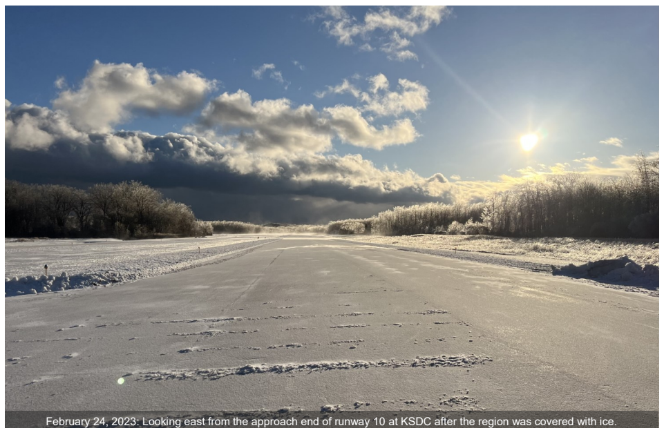
February 24, 2023: Looking east from the approach end of runway 10 at KSDC after the region was covered with ice.
