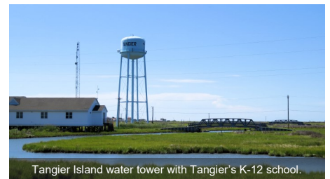
Tangier Island water tower with Tangier's K-12 school.
