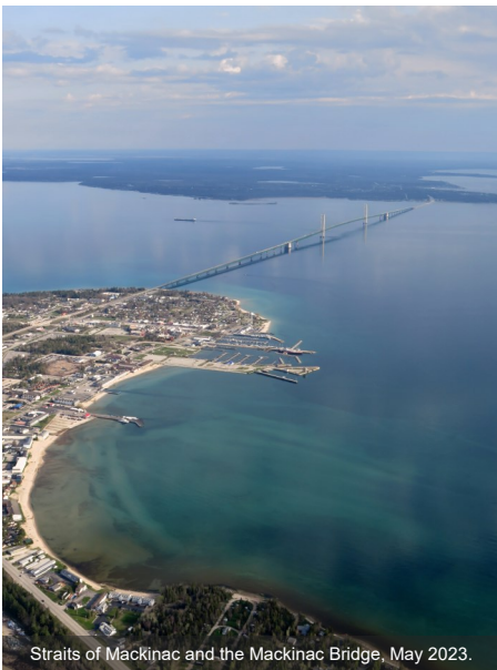
Straits of Mackinac and the Mackinac Bridge, May 2023.
